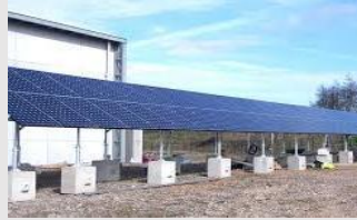
Concrete Pile Total of 4700+ MW
