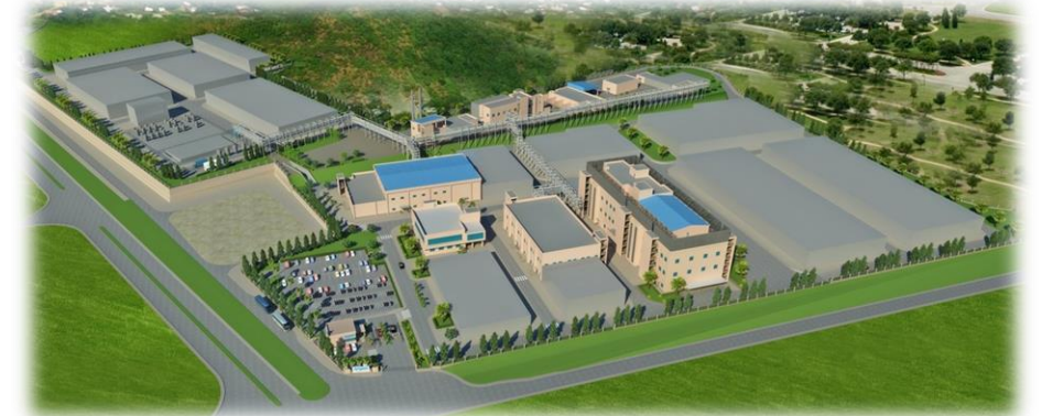
Syngene's API manufacturing facility at Mangaluru
