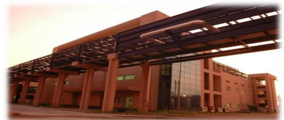
Syngene's USFDA approved manufacturing facility at Bengaluru
