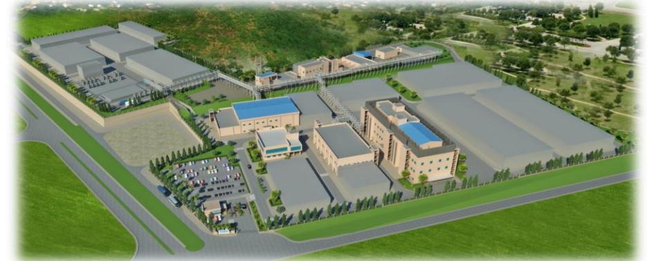
Syngene's API manufacturing facility at Mangaluru
