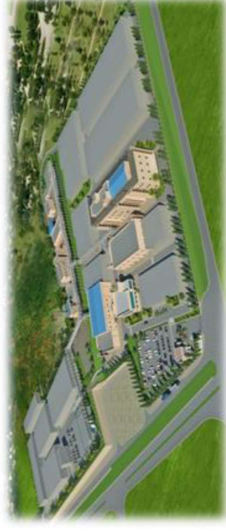
Syngene's API manufacturing facility at Mangaluru
