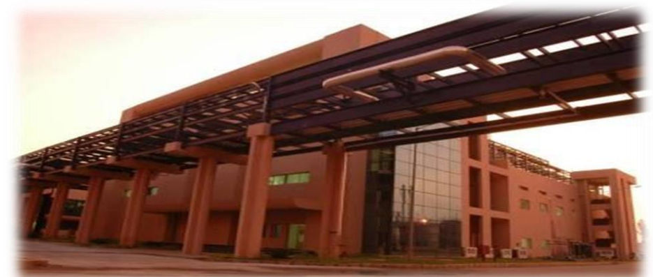
Syngene's USFDA approved manufacturing facility at Bangalore
