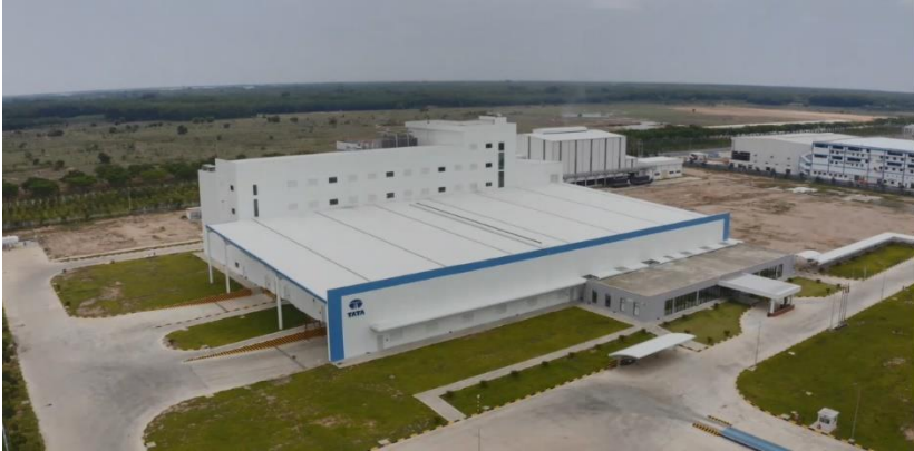
State-of-the-art Freeze-Dried Instant Coffee manufacturing facility in Vietnam with a capacity of 5,000 MT per annum.
