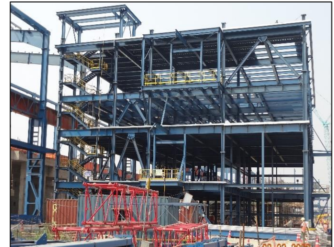
ECR Building of PLTCM
