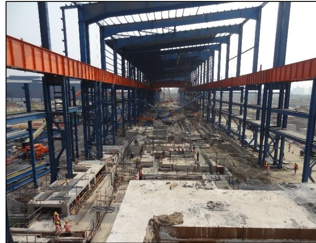
Entry side equipment foundation of PLTCM
