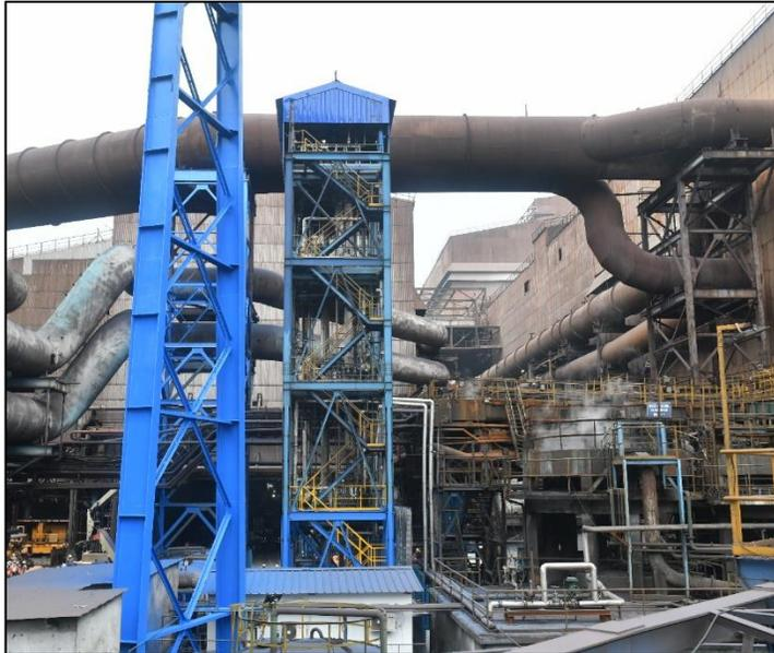
Commissioned 5 TPD CO<sub>2</sub> capture plant at Jamshedpur; first in India by a Steel company to extract CO<sub>2</sub> directly from Blast Furnace gas
