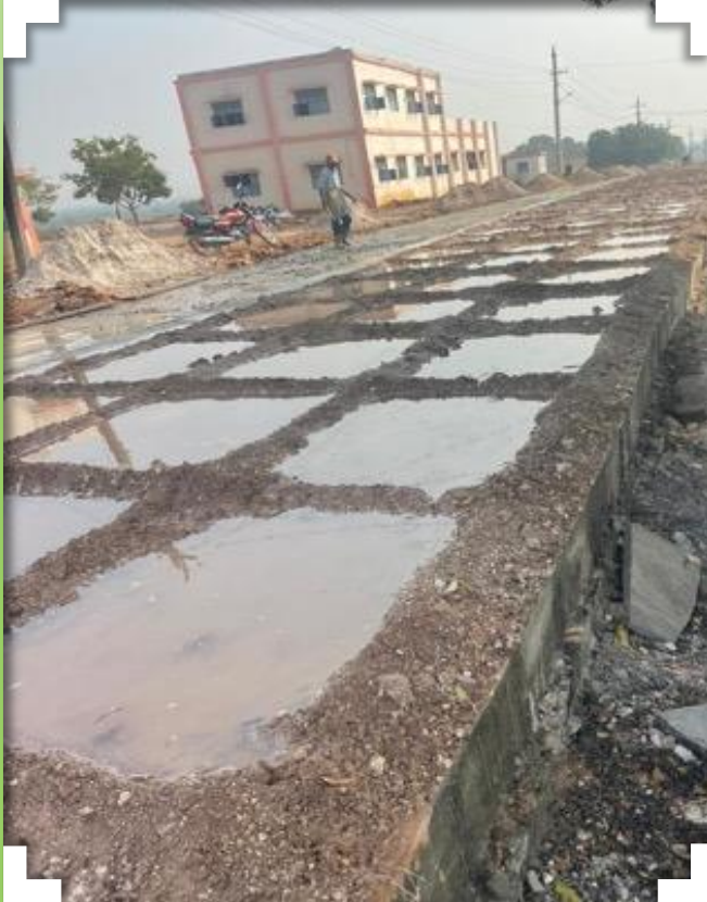
Internal village roads built near Andhra Pradesh Cement Works, Andhra Pradesh
