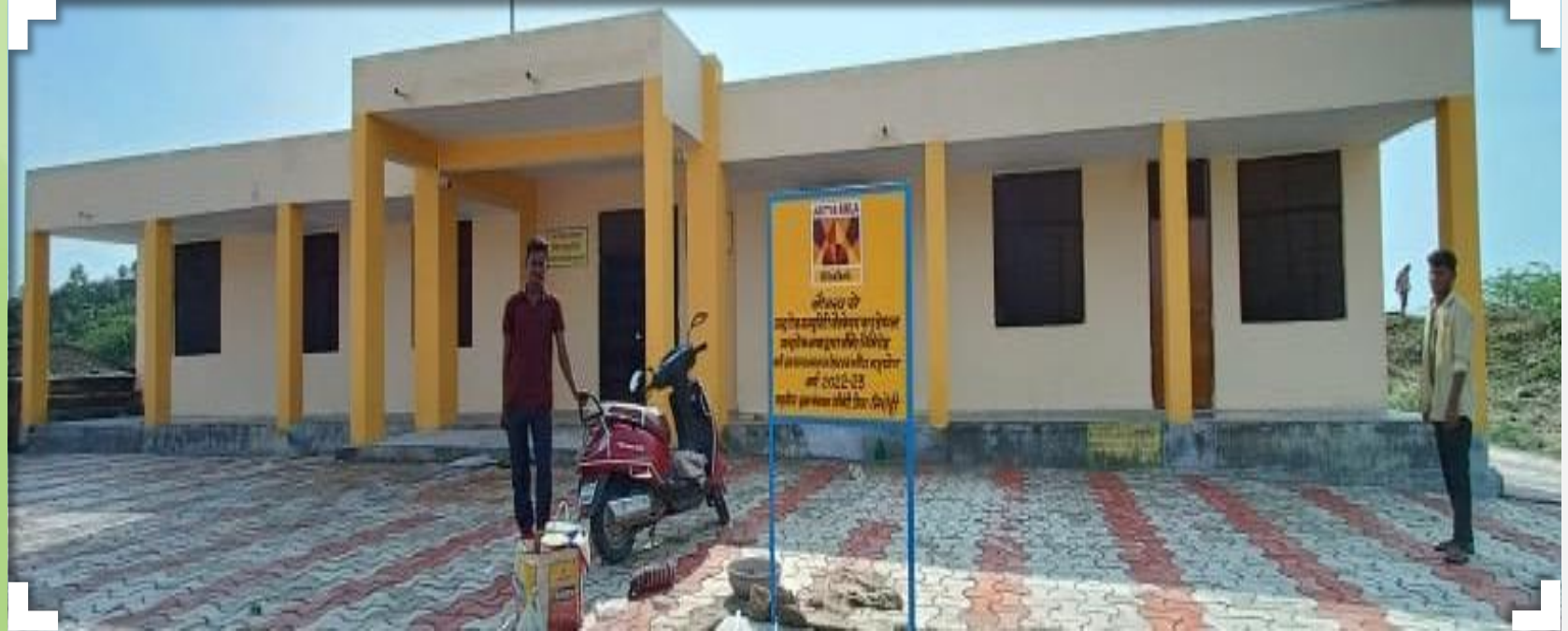
Refurbished community hall for social activities at Nathdwara, Rajasthan
