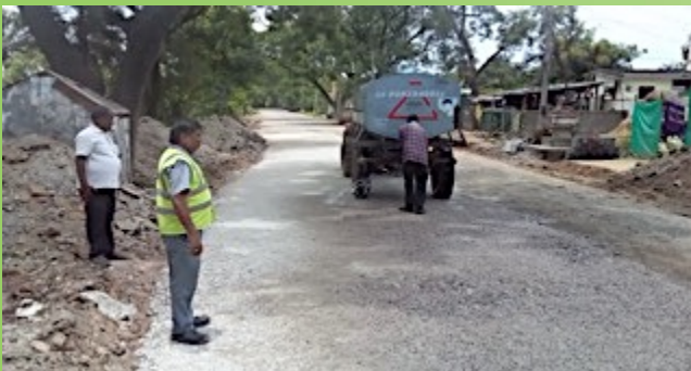
Balaji Cement Works, Andhra Pradesh
