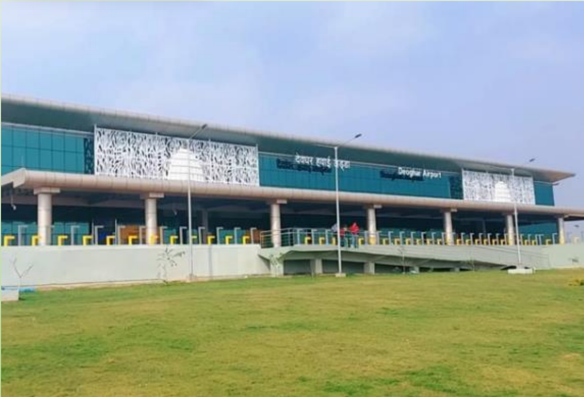
Deoghar Airport, Jharkhand – UltraTech supplied more than 85% of the cement consumed in the project
