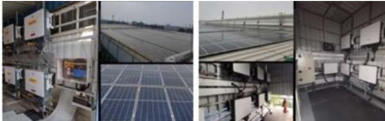
4W Switch Plant Pune
