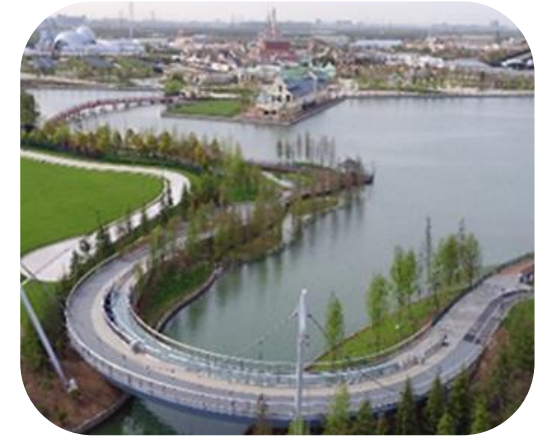
Disneyland, Shanghai, China - Full locked coil, supporting cables
