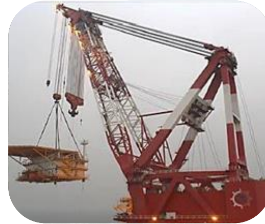
ZPMC, China, Barge Crane - Main & auxiliary hoist rope
