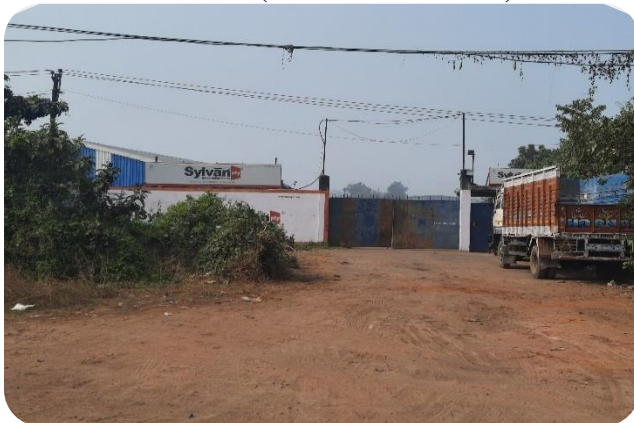
Main Gate (Entrance from NH-2)
