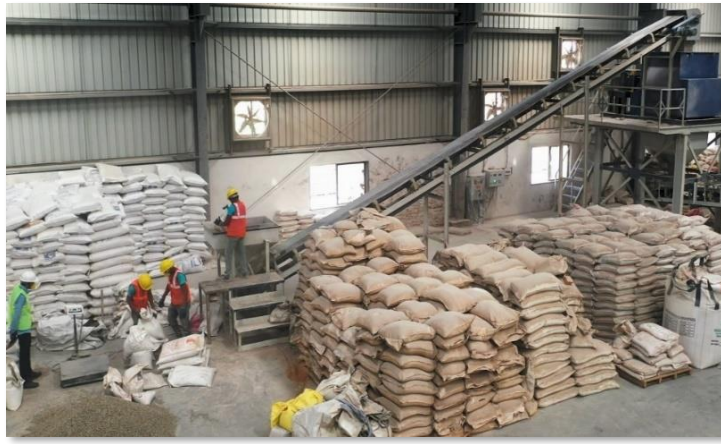
Mixing and packing of Castable
