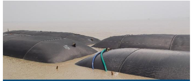
Geotextile Tube for Erosion Control
