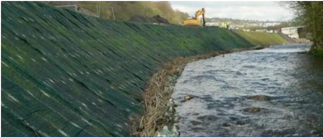
River Bank Protection
