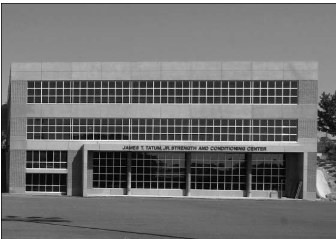
The James T. Tatum Strength and Conditioning Center (bottom) and Lowder Academic Center (top two floors)
