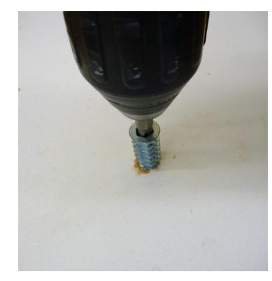
4. Insert all three of the wall anchors in the appropriate locations. Now you are ready to mount the wall charger.
