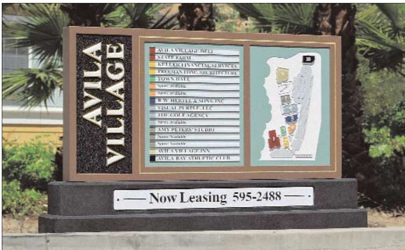
The finished sign installed onto the concrete base. The "For Lease" panel was attached using 3M Dual Lock. A "Welcome to the Village" sign was made to replace the "For Lease" sign when there is full occupancy on the property.
