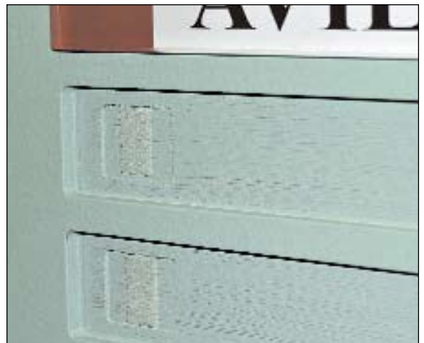
A close-up of the recloseable 3M Dual Lock fastener. It works great for low profile repositioning of elements in outdoor situations. I routed a 3/32" inlay to keep the plaque snug when snapped into place.
