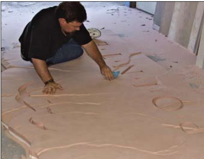
It took me just as much time to hand sand the grinder marks free from the slab.
