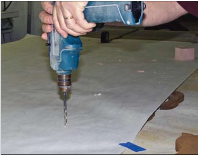
A pattern is laid out and the slab is pre-drilled to accept the all-thread studs for the word "Spyglass".
