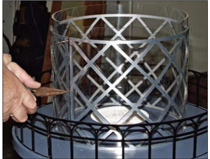
At the back of the lighthouse, the handrail and cylinder shroud were both tied in place with copper wire making for a snug and permanent fit.
