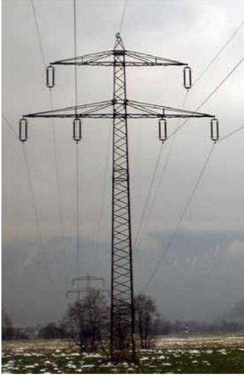
Narrow structures with special requirements for foundations and wind loads
