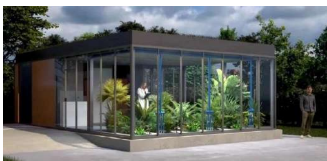
Figure 1. Attractive and compact, this decentralized NBS facility uses Biopolus MNR technology to treat and recycle 50m 3 /day wastewater, with options for energy & organic waste recovery.
