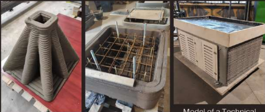
Foundation Footings with Optimized Shape and as Lost Formwork
