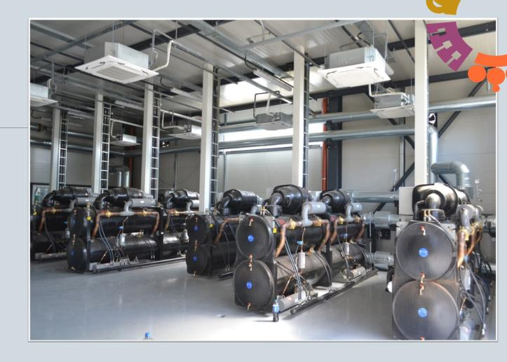
The major element of energy efficiency is given by the use of heat pumps that recover an additional percentage of approx. 40% of geothermal water heat
