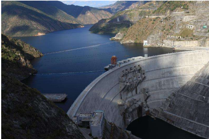
Xiaowan Hydropower Station (4200MW) , 2010
