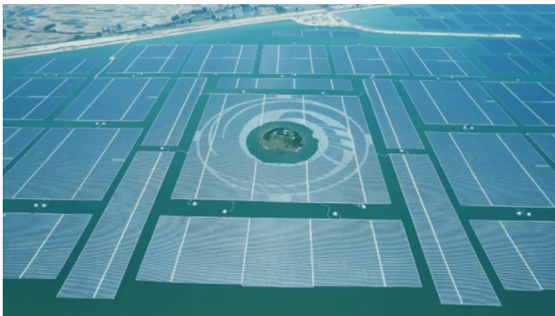
World's Largest 320MW Floating Solar Farm
