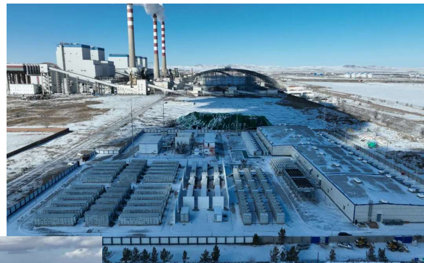
Shangdu Battery Storage Station in China (300MW/600MWh), 2023
