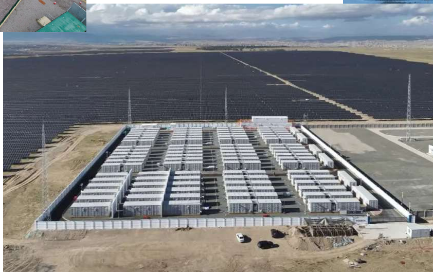
Hainan State Battery Storage Station in China (150MW/600MWh), 2024
