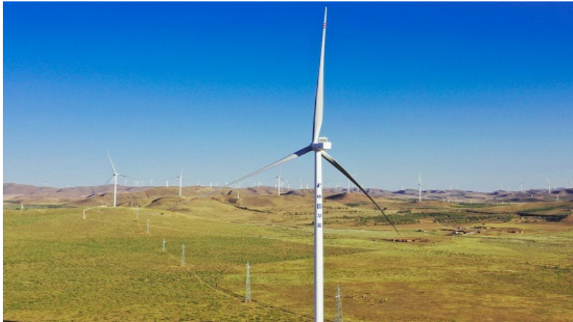
Shangdu 1600MW Wind Farm
