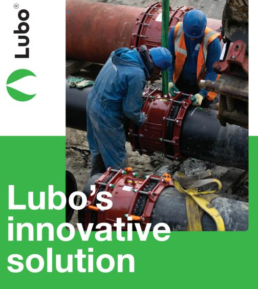
**PFAS-free** assembly for water & infrastructure Assembly has never been this easy. Lubo's fastening materials are ready to use and pre-lubricated with a dry, environmentally friendly lubricant. Prevent cold welding, save time, and cut costs. A smart choice for your projects and our environment.
