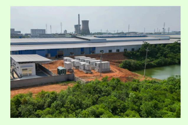
Anfu Eco-Tech, a leading waste management and green technology company in Hunan Province in deploying their **25MWh** energy storage project with five 5MWh energy storage containers
