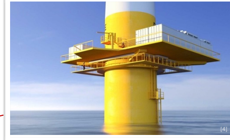
▲ 8 out of 72 Turbines fitted with extended deck for topside electrical equipment and hydraulics
