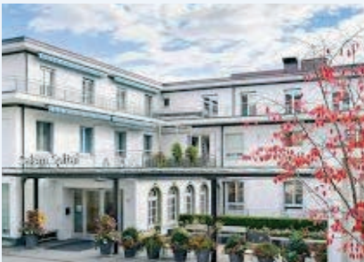
Hirslanden Salem Spital - Bern, Switzerland High Capacity Water Heaters
