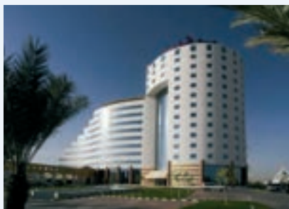
Movenpick Hotel Qassim - Saudi Arabia Electric Water Heaters
