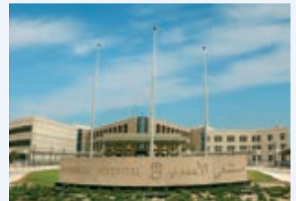
New Ahmadi Hospital - Ahmadi, Kuwait High Capacity Water Heaters
