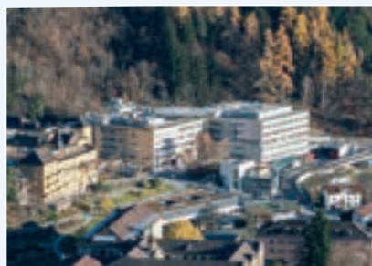
Hospital St. Vinzenz - Zams, Austria High Capacity Water Heaters
