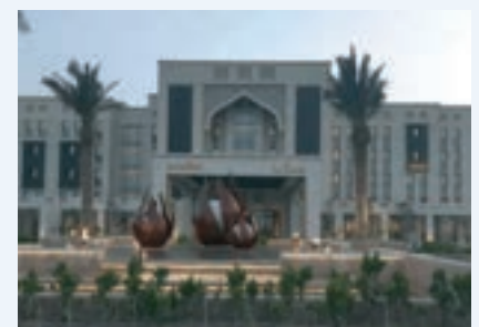
Al Sahel Resort - Bahrain Hot Water Boiler System
