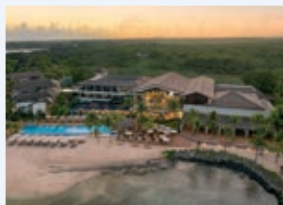
InterContinental Resort - Mauritius Hot Water System
