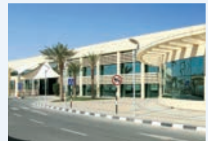
Western District Hospital - Dukhan, Qatar Electric Water Heaters
