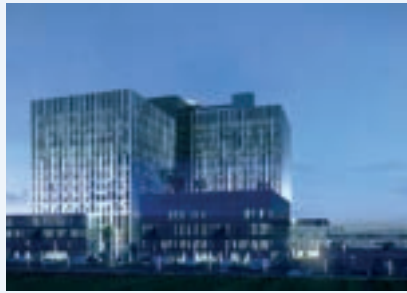
Al Adan Hospital - Hadiya, Kuwait High Capacity Water Heaters
