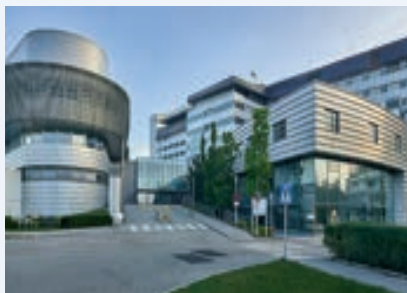
Hospital BHS - Ried, Austria High Capacity Water Heaters
