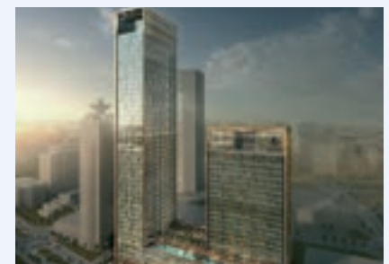
Four Seasons Burj Al Shaya - Kuwait Steam System
