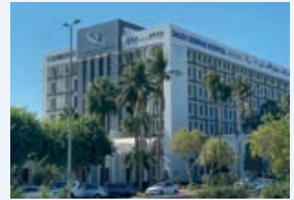
Saudi German Hospital - Jeddah, Saudi Arabia Turnkey Hot Water System
