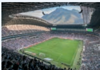
Estadio BBVA Bancomer - Guadalupe, Mexico Turnkey Hot Water System
