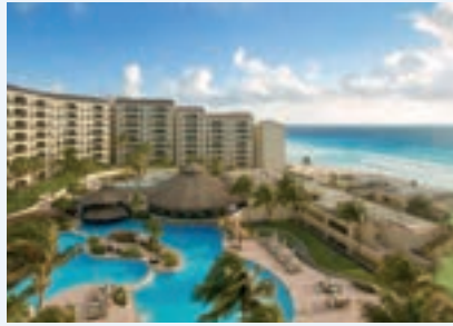
Hotel Emporio Cancun - Mexico Hot Water System & Pool Heating
