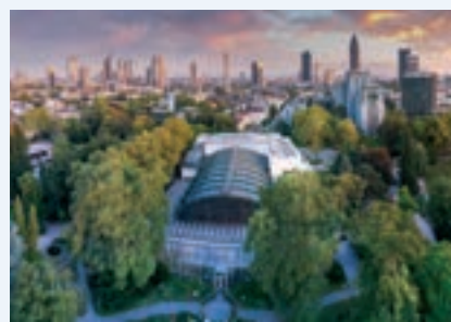
Palm Garden - Frankfurt, Germany High Capacity Water Heaters
