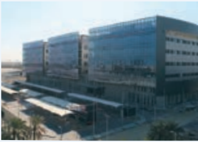
Infectious Disease Hospital - Kuwait Turnkey Hot Water System
