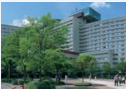
Hospital Klinikum Augsburg - Augsburg, Germany High Capacity Water Heaters
