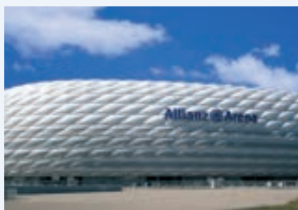
Allianz Arena - Munich, Germany Heat Exchanger
