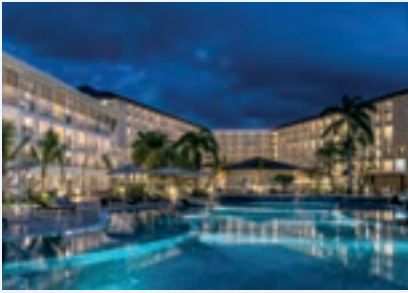
Royalton White Sands Hotel - Jamaica Hot Water / Boiler Package U3 + HE
