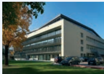
Ferrari School - Innsbruck, Austria High Capacity Water Heaters
