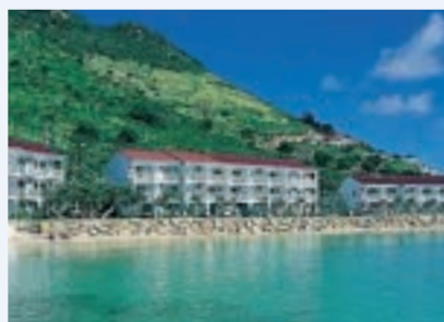
Pelican Resort Club - Simpson Bay, Sint Maarten Hot Water System
