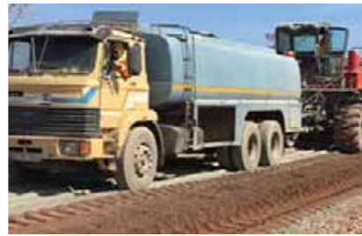
Railway tracks in Turkey
