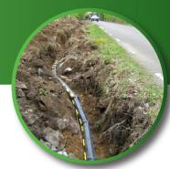
Snipp & Snapp® Hardlock cable protection is produced in diameters from 60-220 mm, including moulded sleeve and three pre-mounted locking clamps in desired colour. The divisible pull-resistant sleeves provides an ideal connection to ensure that the entire line remains fully protected, even over long distances.
