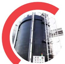
NaOH 50% storage tank with unloading and medium transfer installations – insulated and heated double-walled pipelines with a leak detection system.
