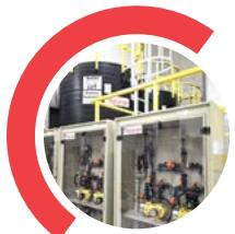
Refuelling, storage (3 tanks, 15 m<sup>3</sup> each) and dosing system for NaOH sodium hydroxide, equipped with the necessary sensors and complete automation controlling the equipment.
