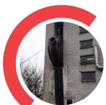
A large-size demineralised water tank with a capacity of 60 m<sup>3</sup> and a height of 9 m, assembled on site from individual cylinder segments.
