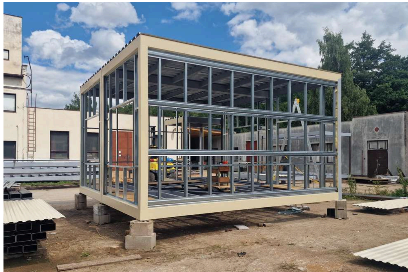
New steel structure
