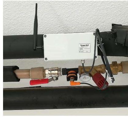
ISURLOG-LR deployed unit remotely monitoring flow and temperature on a hot water distribution network with LoRa comms.
