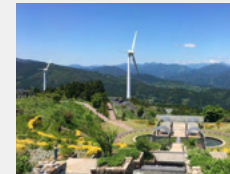
Power generation units monitoring
