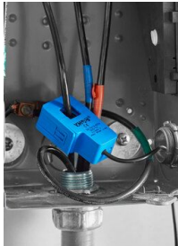
Non-Intrusive Current Sensor in Machine Electrical Panel
