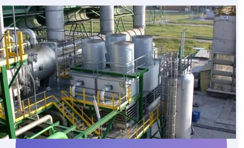
The system is equipped with 1 cogeneration engine of 4.5Wh, 2 boilers of 20 t of steam, 1 photovoltaic system of 600 kW
