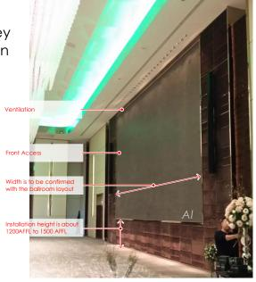
Projection screen and projector shall be designed in detail to avoid clashing with the chandelier. We use 3D model and our BIM system to help the designer to design the spacing and select the right model for projection.
