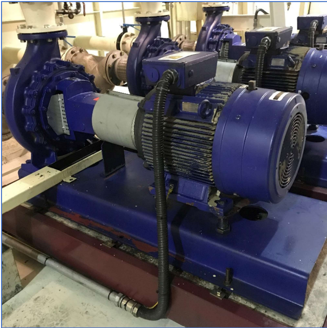
Change of 35mm 2 wiring, wire protection and Siemens switch (before vs. after)
