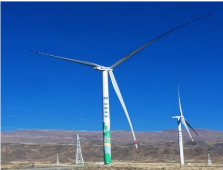
300MW Onshore Wind Farm in Qinghai
