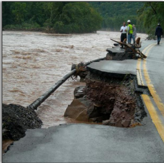
Exposed Petroleum Pipeline Due to Flood
