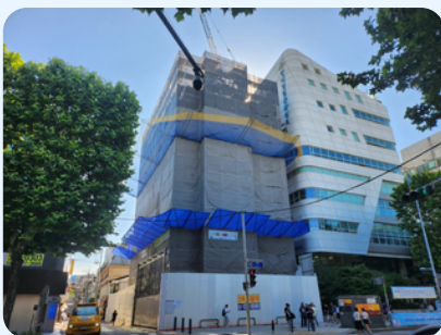
General Construction Co. Suseo·Bangbae PoC Site
