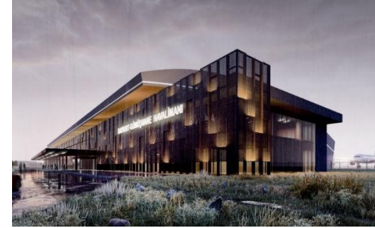
BAYBURT-GÜMÜŞHANE AIRPORT (EPC) 2 MIL. PASS/YEAR 2026
