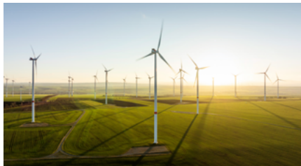
Wind turbines & wind farms
