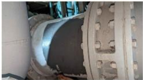
COMPLETED APPLYING PUTTY EVENLY ON THE ENTIRE PIPE SECTION
