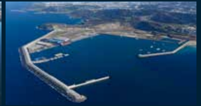
Port of A Coruña
