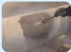
hydro-blasting with non metallic water soluble media
