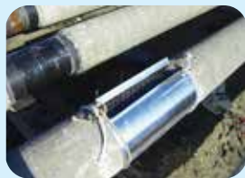
field joint coating
