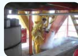
UHPWJ maintenance works
