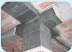
carbon fiber structural reinforcement
