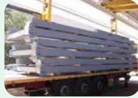
passive fire proofing before erection
