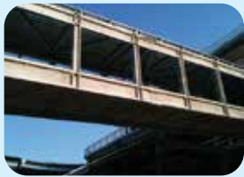
cellulose fire proofing
