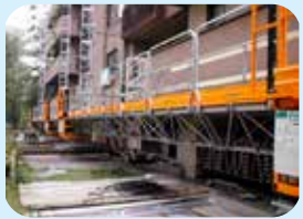
restoration of facades with rampant bridges
