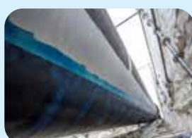
external coating in confined space
