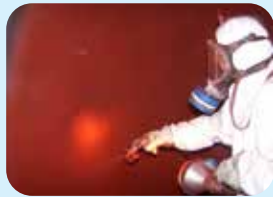
internal lining with food grade coating
