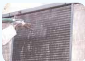
environment friendly coil dry cleaning
