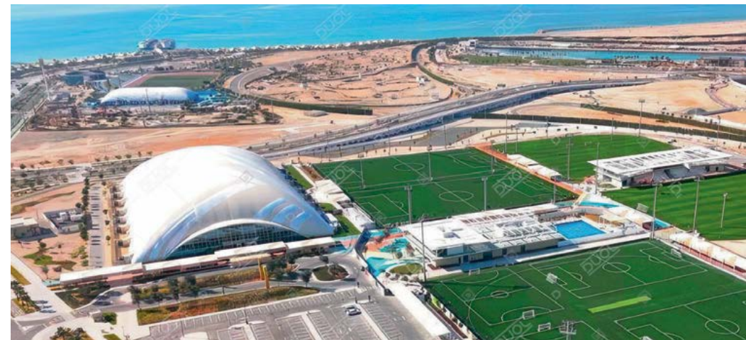
Air dome with AC system and panoramic windows, built in 2023 on Al Hudayriyat Island, Abu Dhabi. Equipped with DUOL ECO Ultra membrane system, it ensures a stable indoor climate (+25°C) at outdoor temperatures up to +55°C. Behind it is our first dome there (2020), reflecting strong client satisfaction and trust in DUOL.
