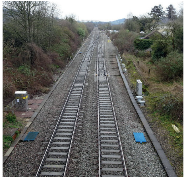
Old Bathampton station (closed in 1966) can be re-opened to provide sustainable travel for residents and support de-congesting roads.
