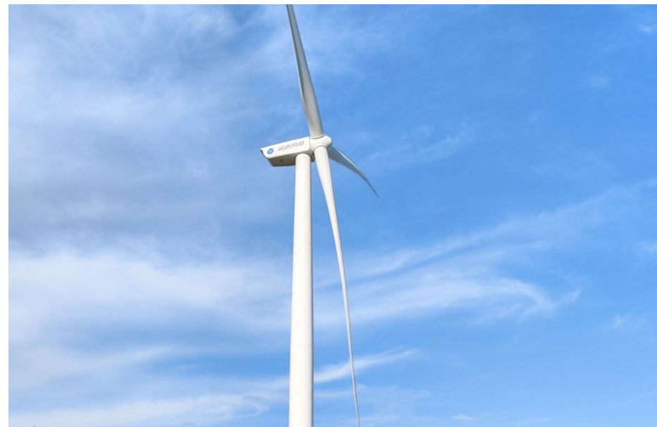
A Wind Farm in Zhangbei, Hebei Grid-forming Technology Application
