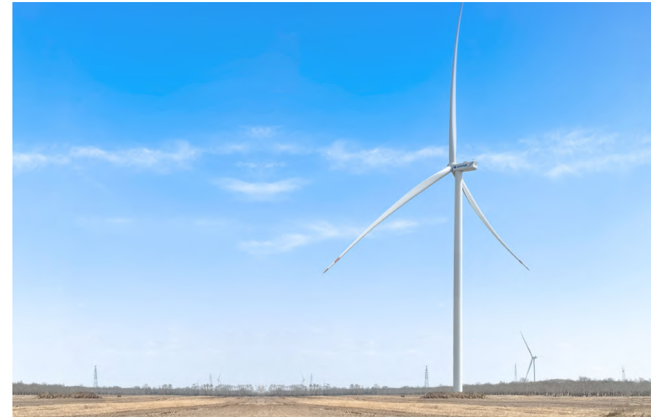
Wind Farm in Zhangbei, Hebei Grid Connection of 1800V Wind Converter
