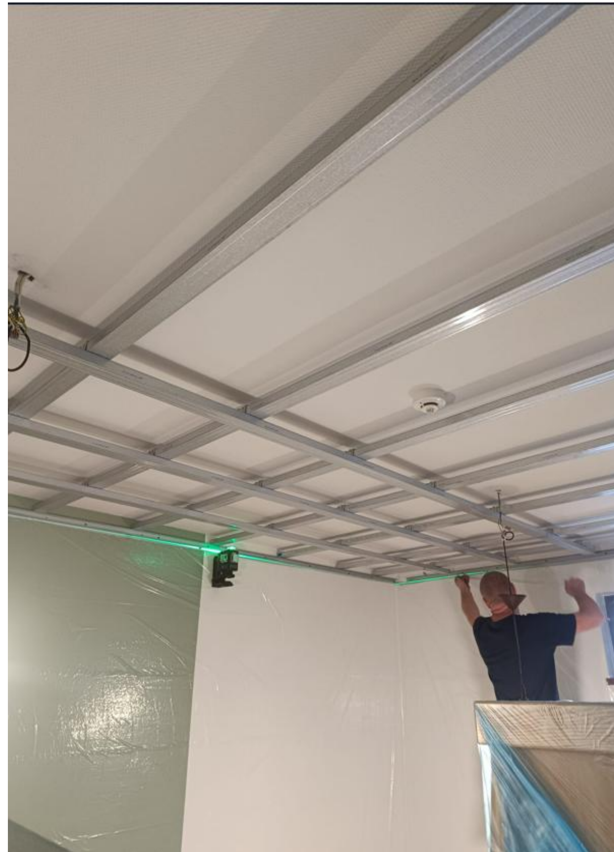
D112 KNAUF 2-level metal profile system or similar
